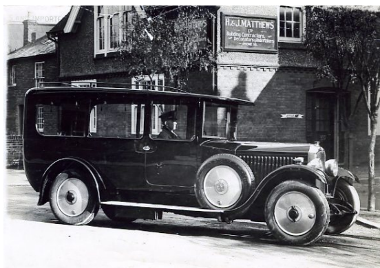
H & J Matthews Ltd, Castle Street Source: BLH&MS (DACHT: BK11887)
